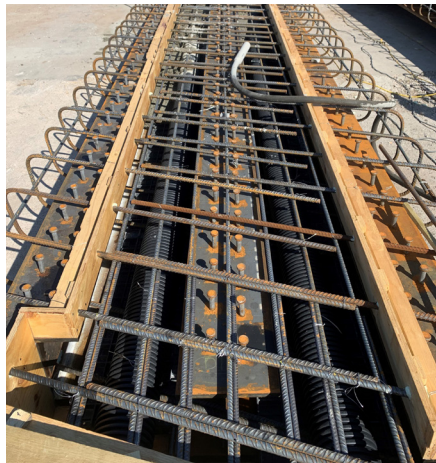
The girders with reinforcement steel installed
