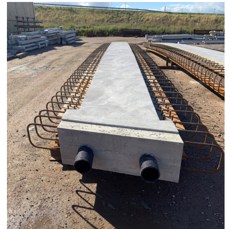
The girders encased in concrete
