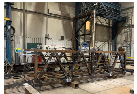
The new walkway being fabricated
