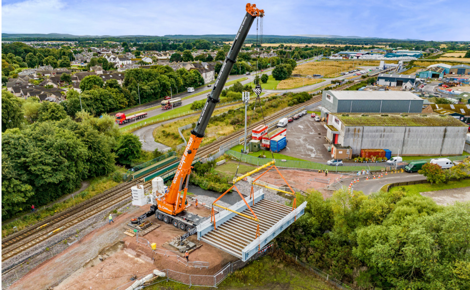
The new bridge being lifted into place at Forres
