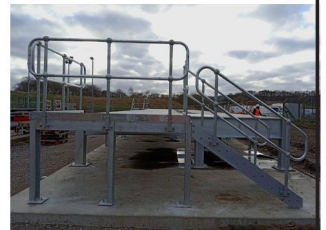
Access steelwork has also formed part of this project
