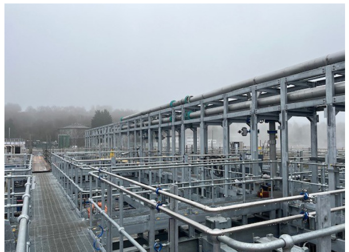
Current progress at the Bolton Wastewater Treatment Plant
